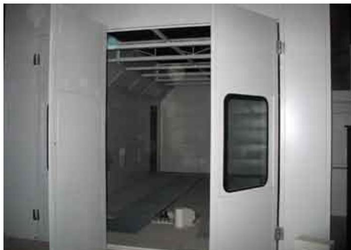
Paint shop personnel are pleased that the physical installation of three new paint booths is nearing completion. Installation of the overhead ducting and electrical work are the next steps in the project. Test runs for the new booths are tentatively scheduled by Christmas.
