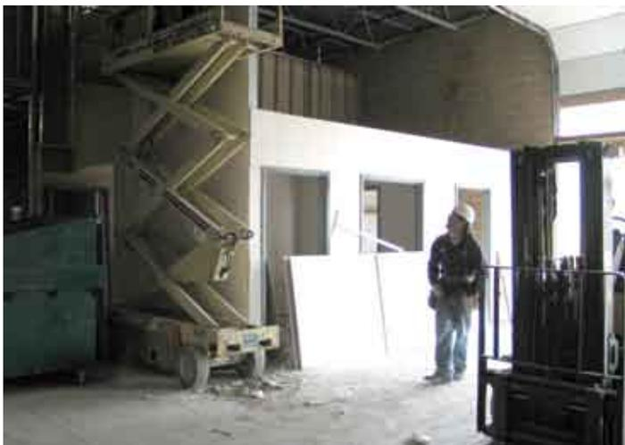
With the majority of work on the outside of Wilson Audio completed and with the change in weather, construction is now focused inside the building. Most of the new offices, including the shipping and receiving offices shown above, have been framed in and sheetrocked.
