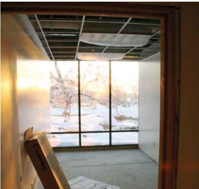
Finish work on the new offices has begun. Oak door frames have been stained and doors will soon be hung. Offices are ready for the final electrical, including the alarm system, before ceiling and carpet are installed.
